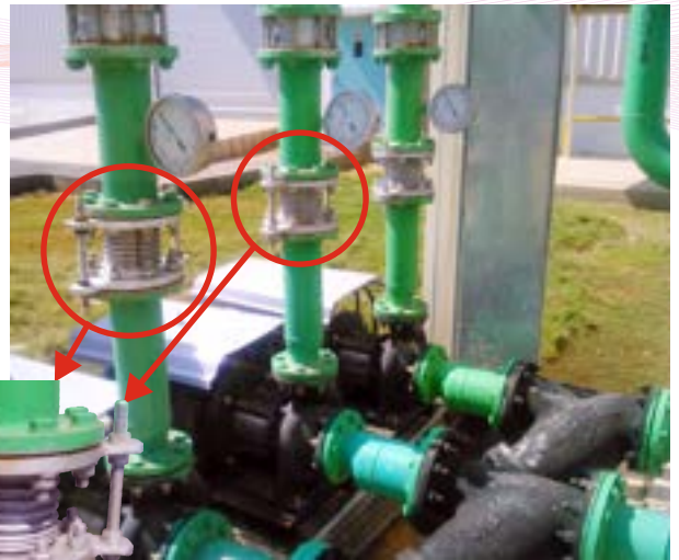
MEJ isolate vibration in Pumps of Honda car Factory
