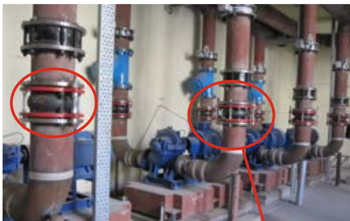
Rubber Expansion Joints at Metro Stations
