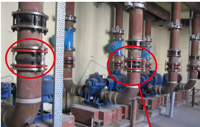
Rubber Expansion Joints at Metro Stations
