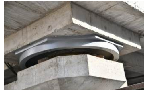
Special Pendulum Isolators with Fuse for over travel protection
