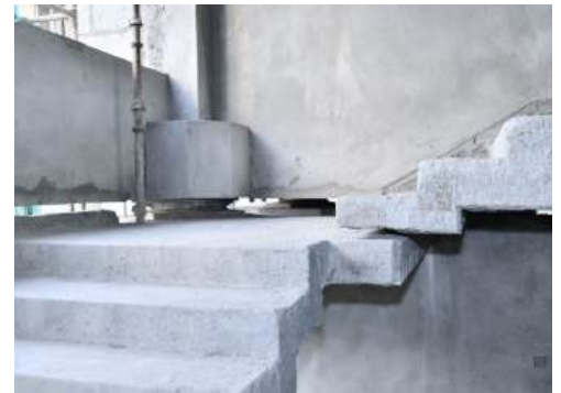
Staircase Isolation for uninterrupted staircase usage during and after an earthquake
